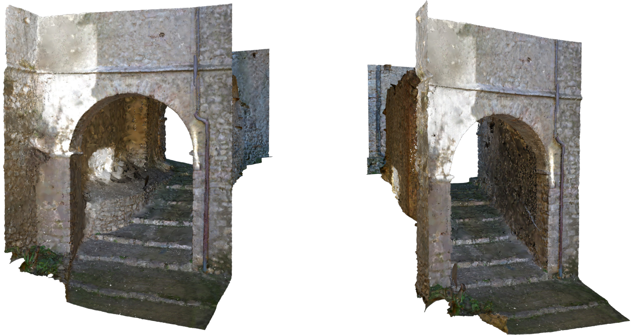
Figure 27. 3D Multi-View Reconstruction result: A scene with a stone staircase. # Face: 353K, Time: 36 min.
