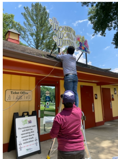
Figure 1: Installing free WiFi at Watkins Regional Park in Covid-19 .
